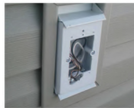
EXAMPLE OF FLASHING WITH END-DAM
